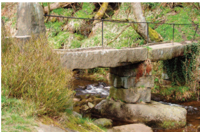
Stone clapper bridge at Hebble Hole
